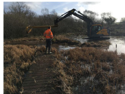
Landmarc contractors clearing vegetation from a Breney pond. Photo: Séan O'Hea
